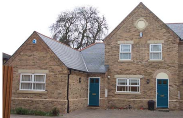
A rare example of a small scheme containing a mix of types and sizes of new homes, and contributing to the need for smaller properties (Oriel Court, St.Ives).
